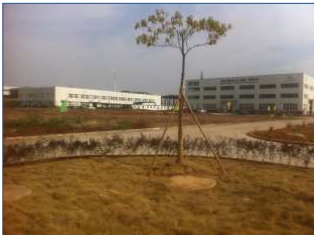
November 2012 – Ground Breaking
